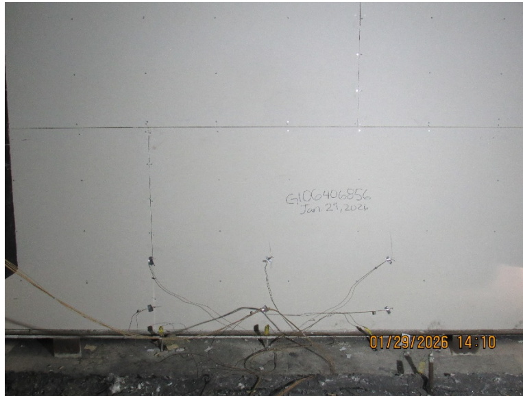
Photo No. 11 Second floor Prior to testing
