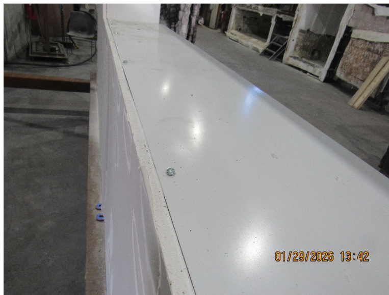
Photo No. 10 Flashing installed by client
